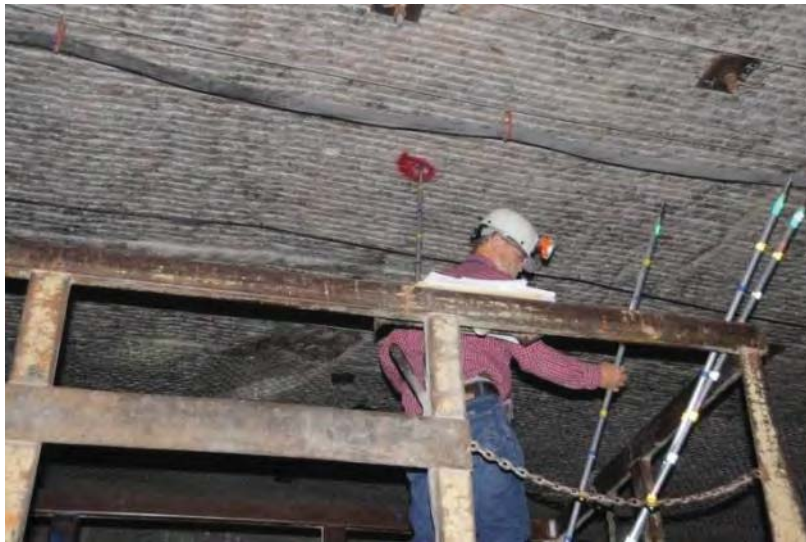
Figure 1. Taking Fracture Measurement at Observation Hole OH1018
